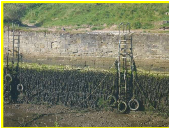
Wall on west side of harbour (/4401C04)
