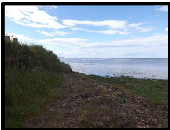
1401/C02 – 2016 at corner to South Low Channel.
