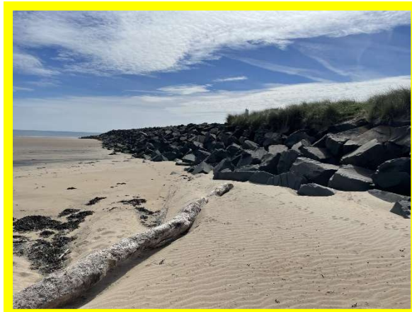
Rock armourstones on north face of North Pier (/3001C01)
