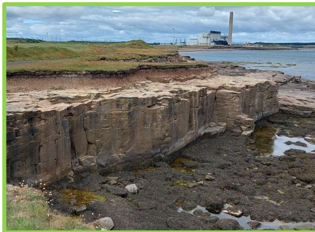
Currently relatively stable cliffs around Beacon Point (/3501C11)
