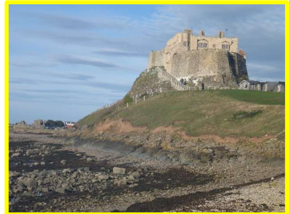
Cliff below castle east of erosion matting (/4901c12).
