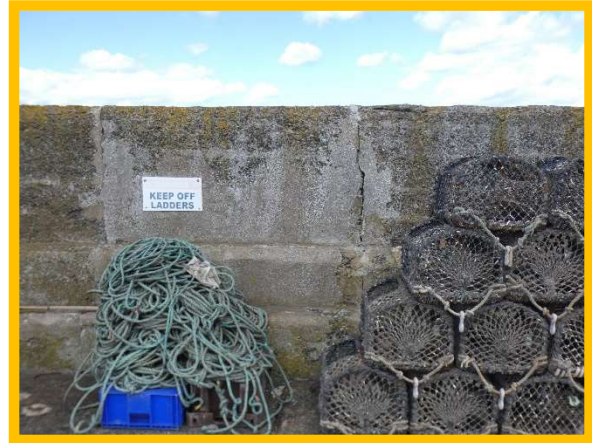
2201C03 Inside face (crest wall) at crack
