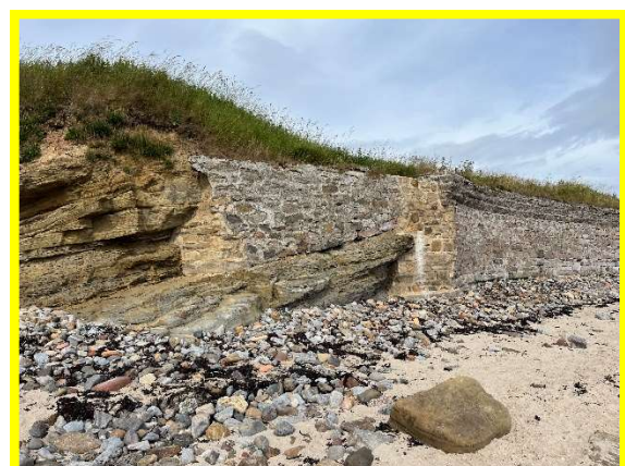
Masonry blockwork wall repaired in 2022 (1701C25)
