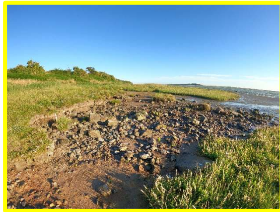
1401C21 – Evidence of salt marsh erosion in Budle Bay
