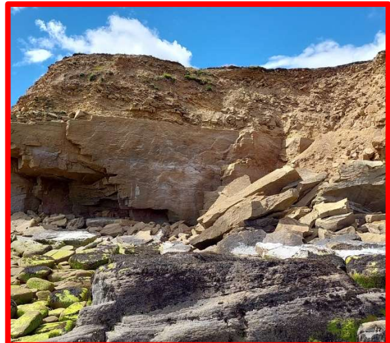
Active sections of Hawks Cliff (/3701C02)
