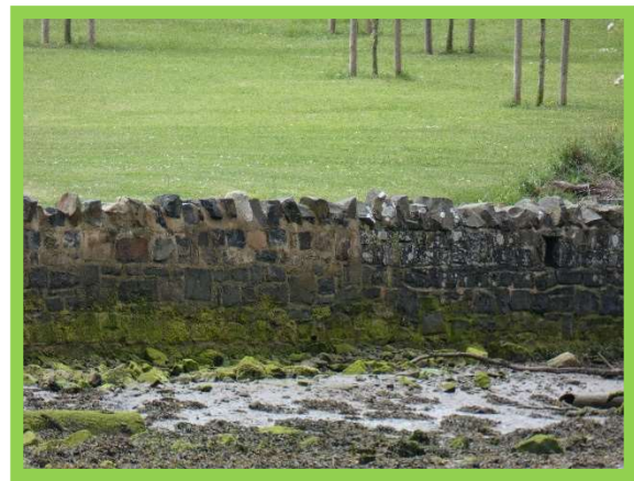
1501/C02 – Wall to new development.
