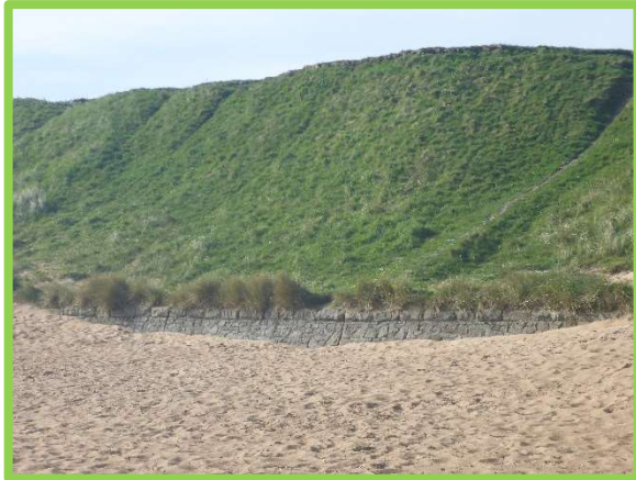
Northern wall in good condition (/4401C01)
