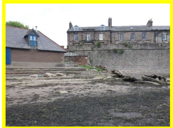
Wall in fair overall condition (/0801C05)
