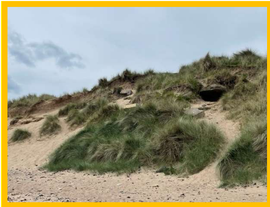
Dunes slumping, exposing concrete rubble (/3101C12)
