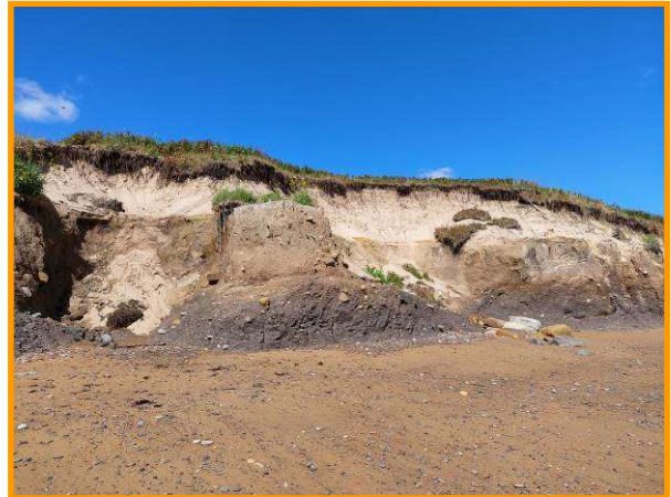
Slumps on Cliff (/3401C01)
