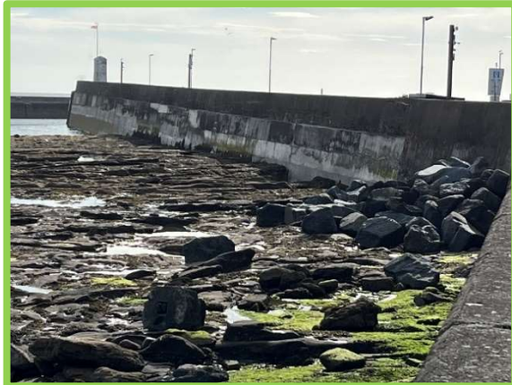
Rock armour wave reduction and Repaired outer wall 1701C06 & 1701C07
