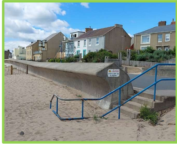
High beach levels in central sections of Newbiggin Bay (/3601C07)
