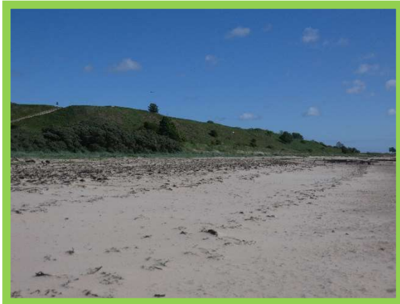
2701/C06 northern, concrete blocks buried.
