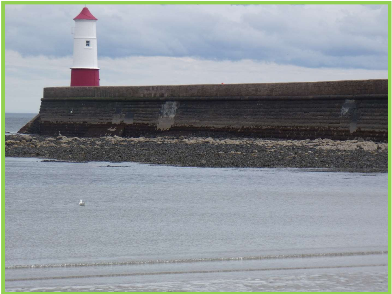
Berwick Pier in good overall condition following refurbishment in 2012/13 (/0701C14 & C15)
