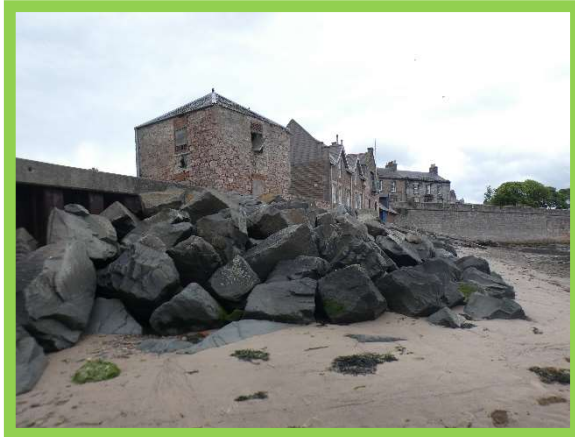
Rock revetment in good overall condition (/0801C04)
