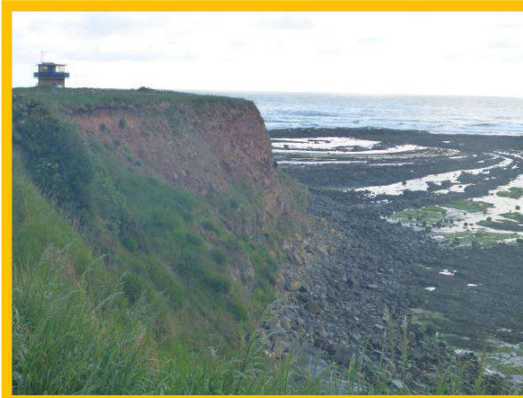
Slumping cliffs along Magdalene Fields Golf Course (/0701C12) 2020
