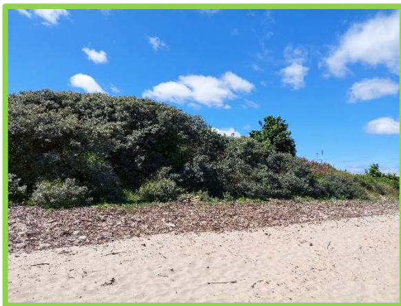
Accumulation of sand at the toe of the cliff (/3801C02).
