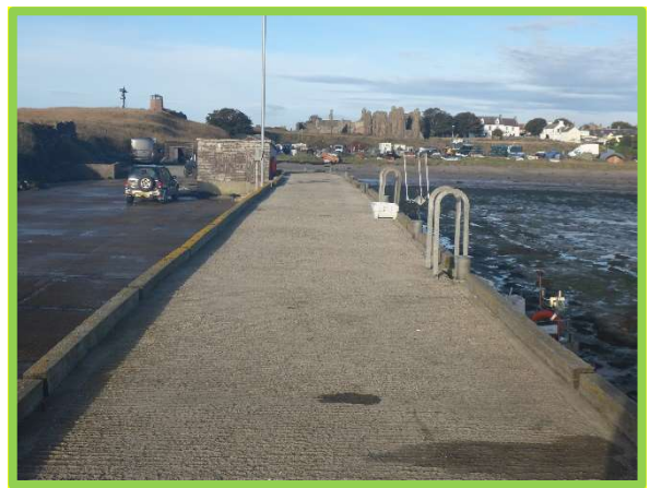
Improvement works to harbour pier (/4901c09)
