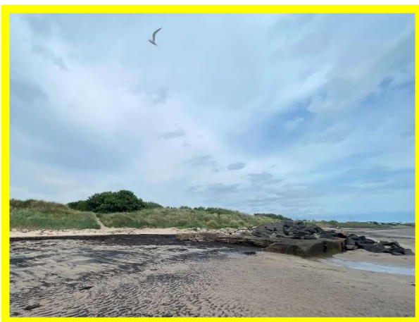
Rock revetment in fair condition (/3201C05) around poor but functional outfall
