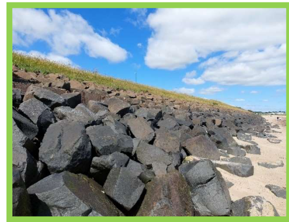
Rock revetment protecting former foundry site (/3901C05)
