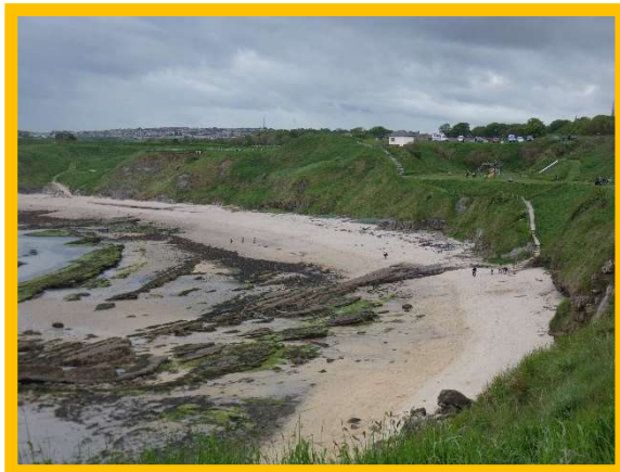
General view of condition across bay (/0701C06 to C10) 2022
