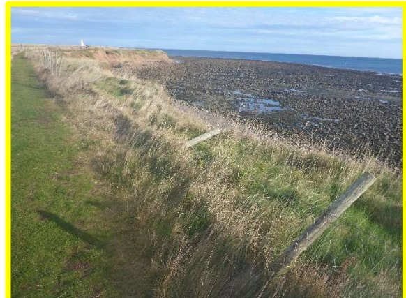
Erosion of soft cliffs remains an ongoing process (/5001c04) and fencing needs re-erecting.
