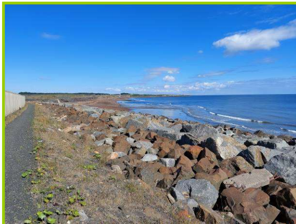
Rock revetment north extension (/3401C07)
