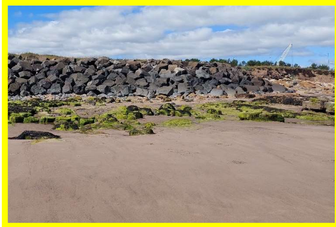
Rock outcrops protecting the north end revetment toe (/4001C01)
