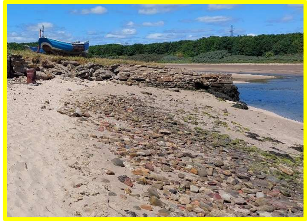
Wansbeck Boat Club retaining wall (/3801C02)
