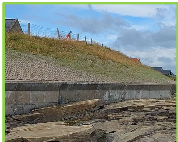
Low concrete wall and interlocking concrete unit revetment at Cresswell (/3201C19)
