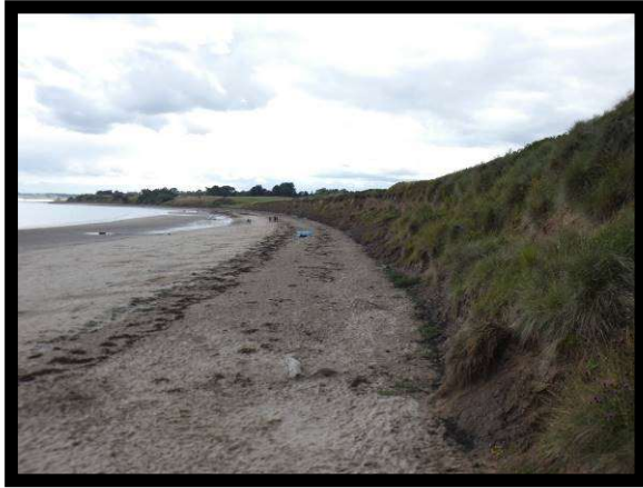
2701/C01 Eroding cliff to golf course 2020
