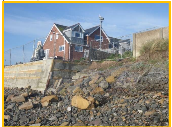
Tie-in section of wall at failing gabions further protected by 2022 (/4201C04)
