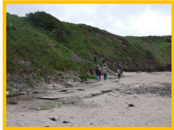
Slumping in cliffs at Greens' Haven (/0701C06) 2022
