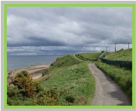
1101/c01 general position of railway line in relation to cliff and coastal slope
