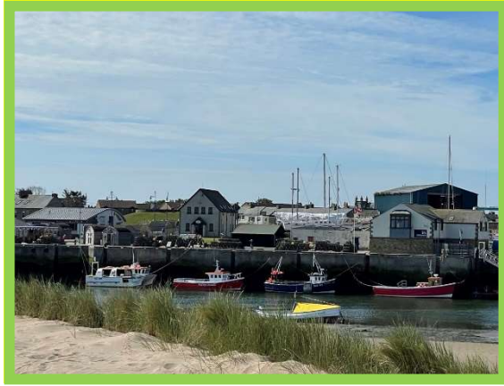
Quay wall in good overall condition (/3001C05)
