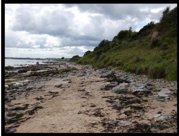
2701/C04 slope remains relatively stable but lower beach with slight erosion 2020.
