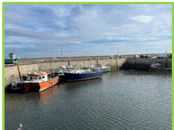
Inner face to North Pier 1701C11
