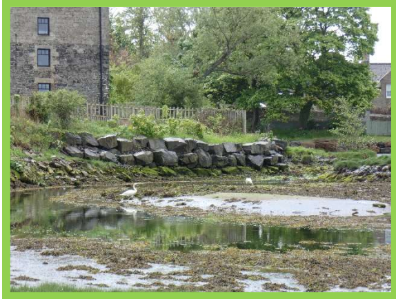
1501/C03 – rock wall to Warren Mill.
