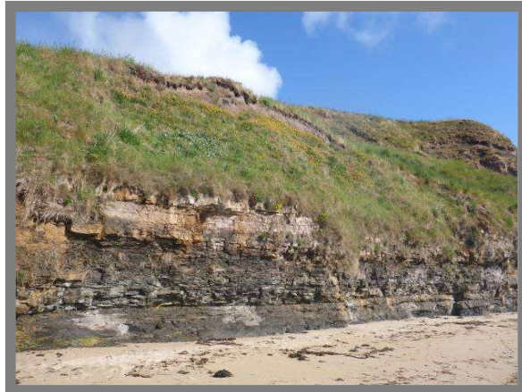
Slumping in cliffs at Green's Haven (/0701C06) 2020
