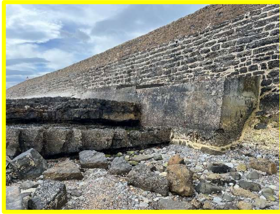
Repaired undermining of seawall at Beadnell North (Nacker's Hole) (1701C36)
