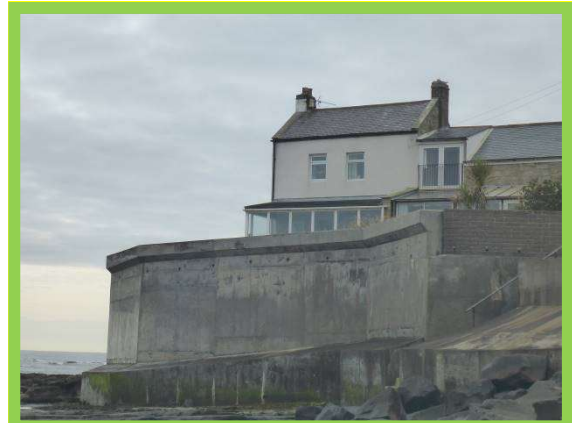
Substantial seawall in overall good condition (/3101C07)
