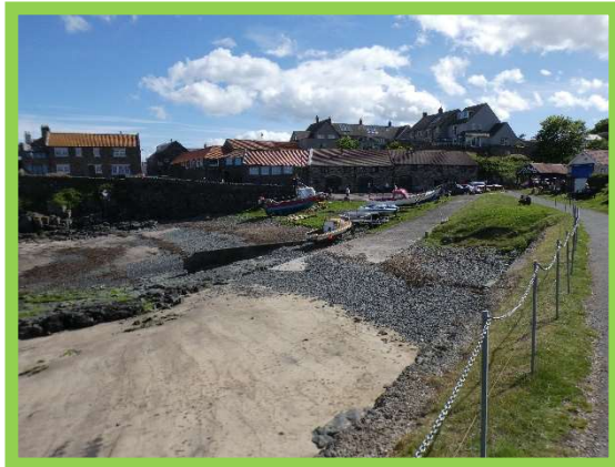
2201/C07 Slipway no change
