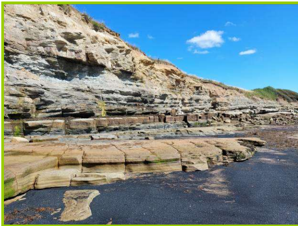
Relatively stable rock cliffs at northern end of Lynemouth Bay (/3301C02)
