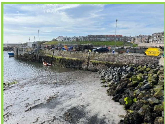
Inner face of the Inner Pier 1701C10
