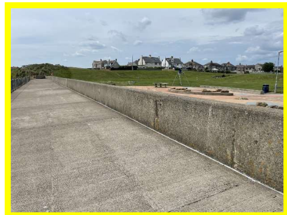
Some staining of the back wall (/3101C05)
