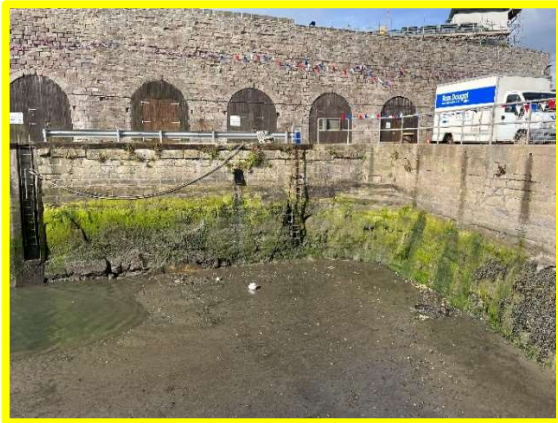
Masonry wall in fair condition 1701C13
