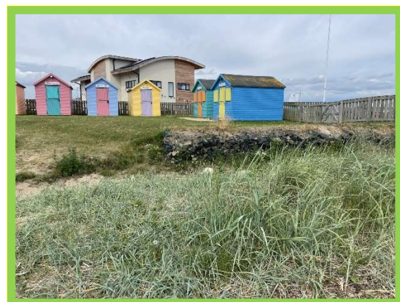
Gabions fronting beach huts (/3001C08)
