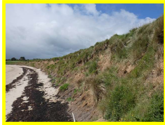
2701/C01 further cliff slumping, with minor erosion at the toe 2022.
