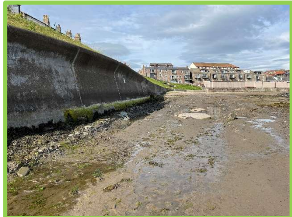
Wall and slope in good condition (1701C18)
