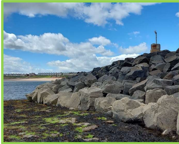
North breakwater in Newbiggin Bay in overall good condition (/3601C14)
