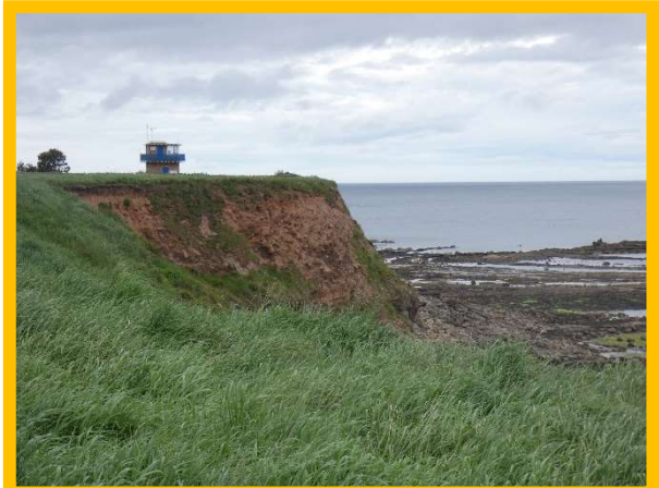
Slumping cliffs along Magdalene Fields Golf Course (/0701C12) 2022
