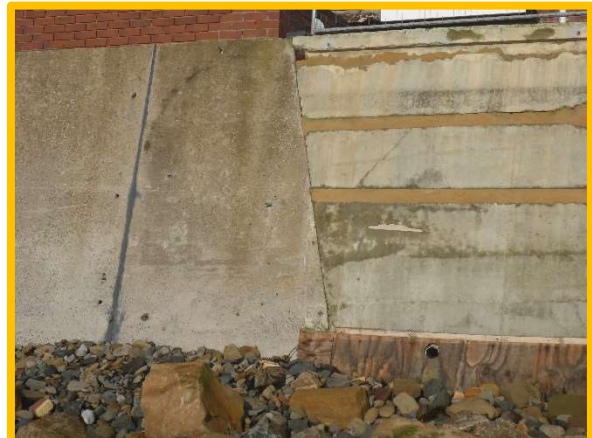
Interface of original and extended sea walls (/4201C04)
