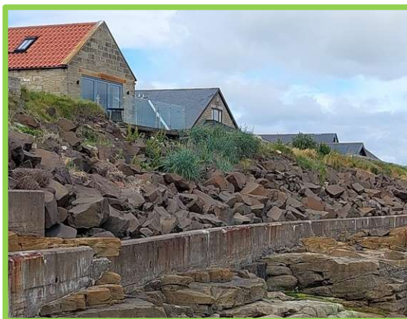
Low concrete wall and rock revetment at Cresswell (/3201C18)
