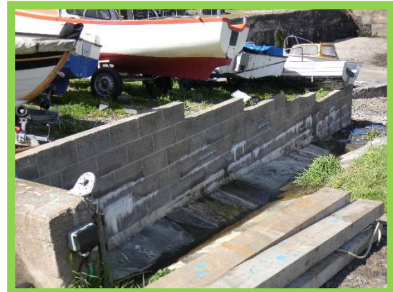
2201/C06 Blockwork wall
