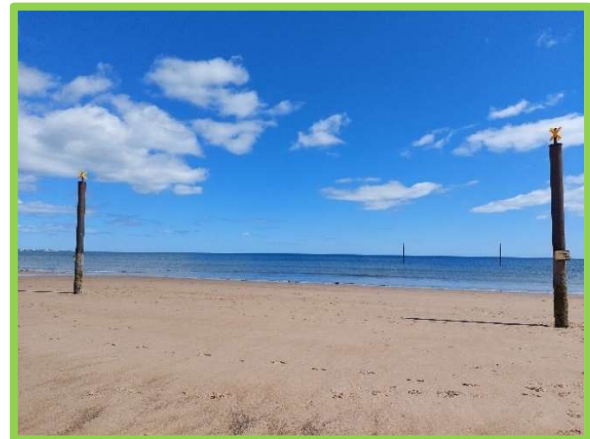
BODF cable landfall signposts (/3901C04)
