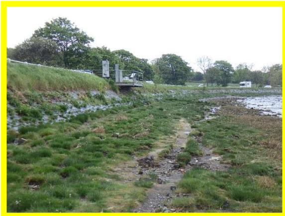
1501/C04 – heavily vegetated revetment
