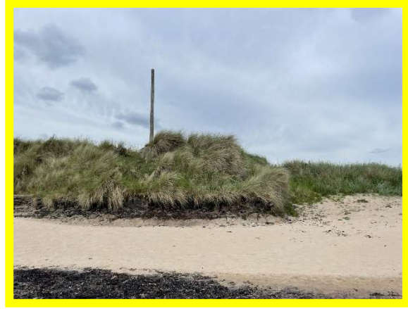
Telegraph marker pole becoming undermined at base through erosion (/3201C07)
