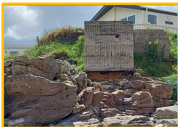
Southern concrete pill box perched on rock ledge (/3501C07)
