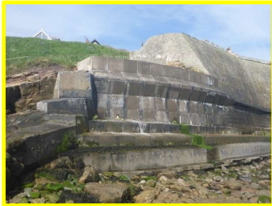
Short length of tie-in sea wall (/4401C16)
