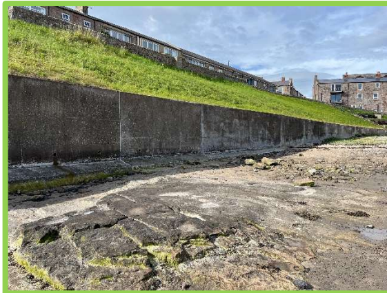
Wall and slope in good condition (1701C17)
