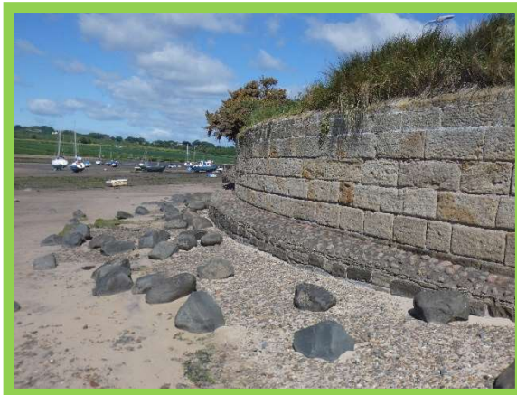
2801/C02 Masonry wall with concrete and cobble toe apron. Little change.
