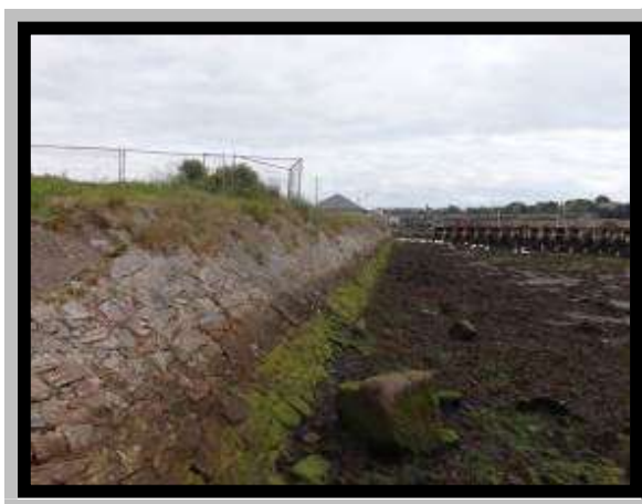
Masonry revetment 901c04 at northern end -2016.
