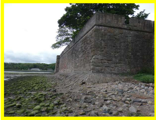
Berwick's historic town walls in good overall condition (/0801C06)
