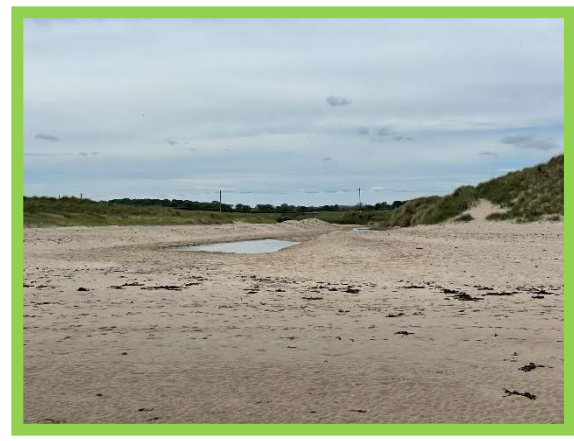
Evidence of excavation works to maintain a channel for the Creswell Northumberland Wildlife Trust pond. (/3201C16)
