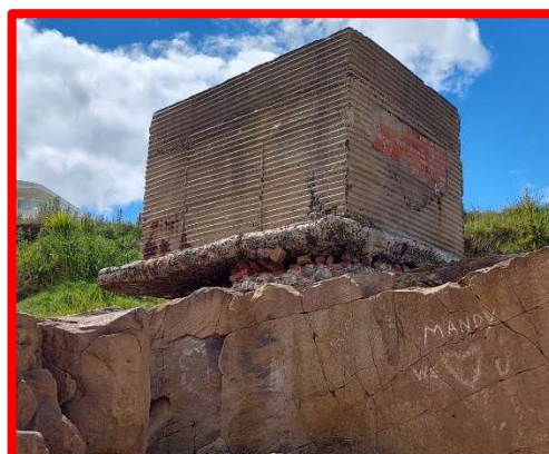
Northern concrete pill box perched on rock ledge (/3501C07)
