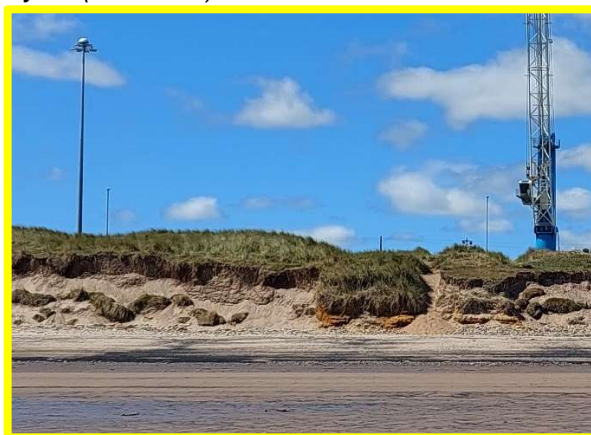
Waterline near the toe of the cliff (/3901C04)
