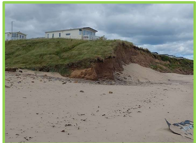
Start of embankment (/3801C01)
