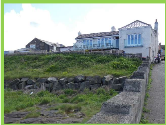
2201/C12 rock revetment at toe of slope
