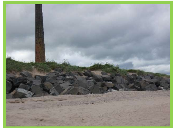
1001 c01 – showing exposure of rock armour 2022
