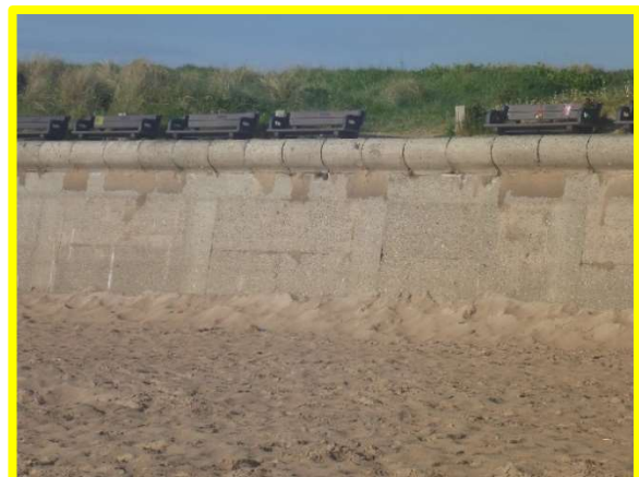
Sea wall fronting southern end of Blyth promenade (/4201C08)
