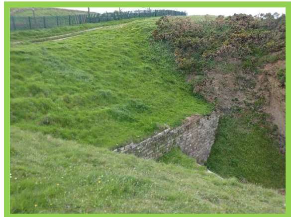
1101/c01 Short section of infill upper slope wall.
