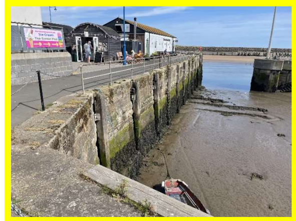
Dock basin in fair overall condition (/3001C06)
