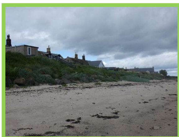
2601/C03 New rock revetment toe (2016) well vegetated.
