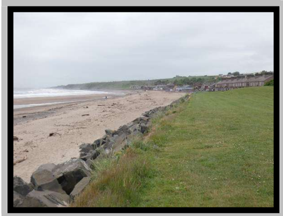
1001 c01 – 2018 showing increased beach width with groyne buried.
