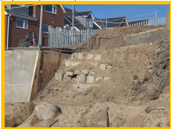
Tie-in section of wall at failing gabions under construction in 2020 (/4201C04)
