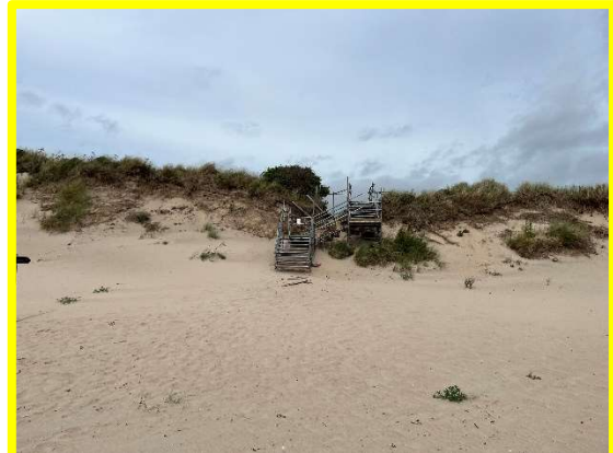
Access steps to connect beach to Long Nanny Bridge (1901C01)
