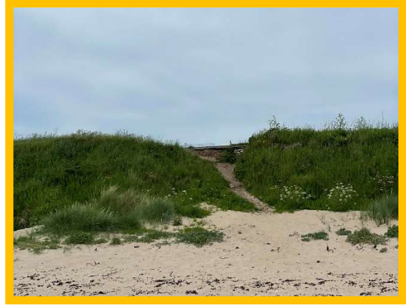
Terminal erosion beyond end of defended section of dune resulting in cut back to road (/3201C14)
