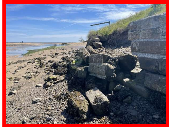
Collapsed section of wall at Church Hill with erosion of the land behind (/2801C13)
