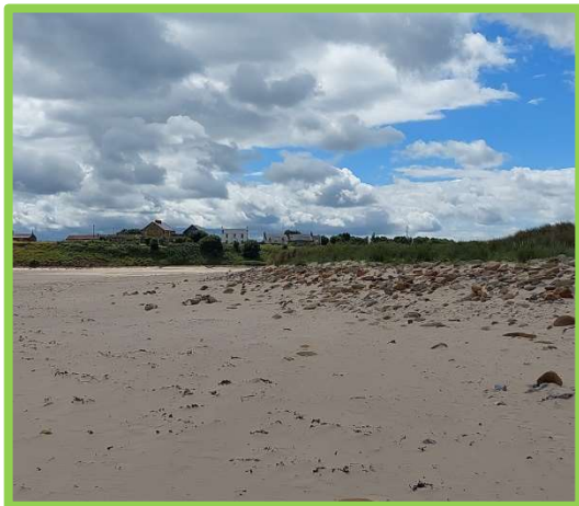
Sand accumulating at the River Wansbeck mouth embankment. (/3801C01)
