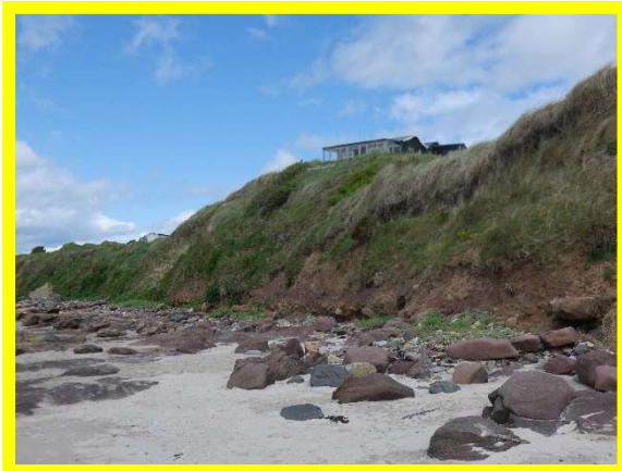
2601/C08 continuing erosion
