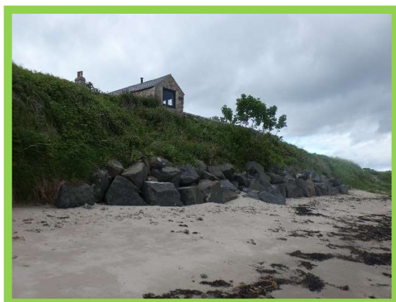
2601/C01 local rock revetment, higher upper beach.
