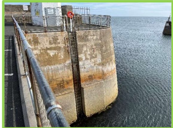
Pier head appeared in good condition 1701C08
