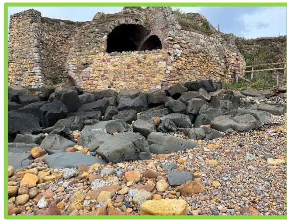
Rock revetment in good condition (1701C46)
