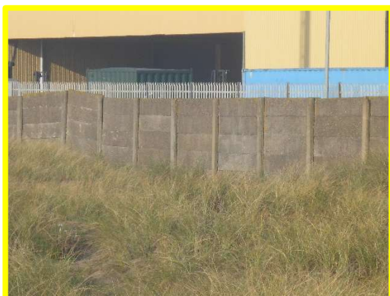
Concrete boundary wall (/4201C11)
