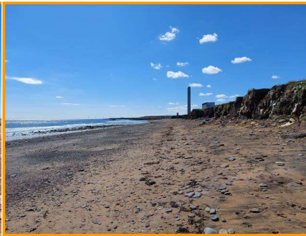
Rapidly eroding colliery spoil beach south of River Lyne leading to erosion of backing man-made cliffs, releasing colliery spoil (and by the river mouth, refuse) to the foreshore (/3401C05)
