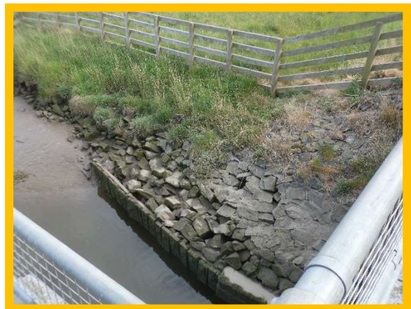
1401/ C01, 2020 view of entrance channel. .
