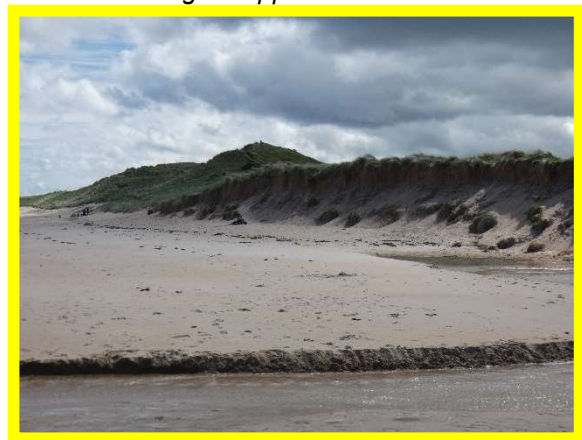
2001C04 2022 local but significant erosion due to configuration of the outfall channel
