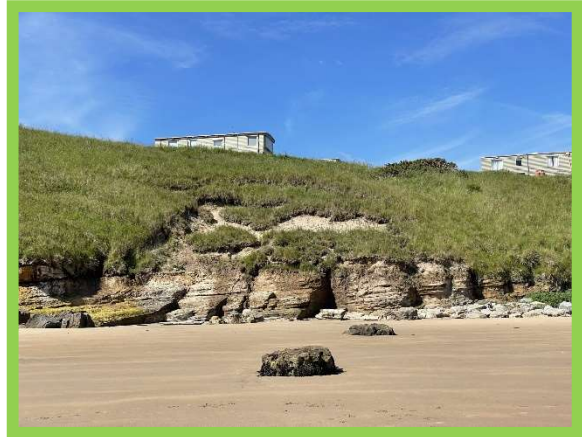
Localised slip at Birling Carrs (2901C02)
