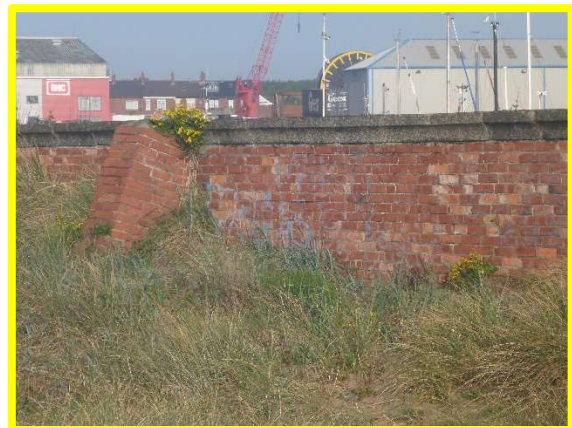
Brick boundary wall to rear of dunes (/4201C10)
