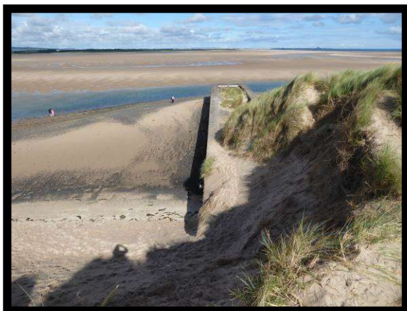
1501/C06 – South face and core of Jetty 2020
