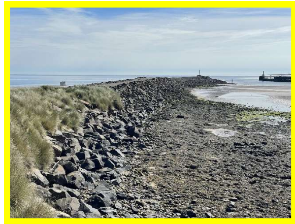
Rock armourstones on south face of North Pier (/3001C03)
