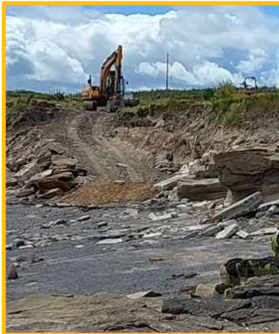
Haul access to the rocky foreshore at the cliff toe (/3701C01)
