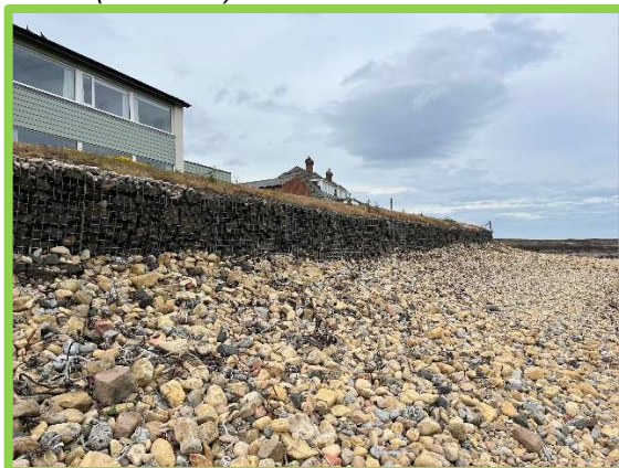
New gabion basket wall in good condition. (1701C41)
