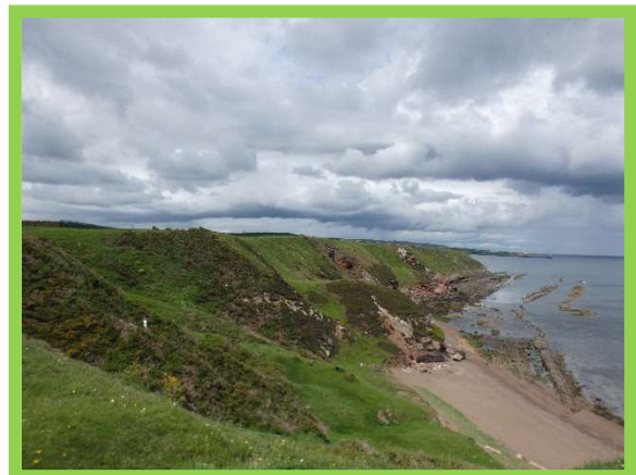
1101/c01 general view of cliffs and beach to north of Sea House 2022.
