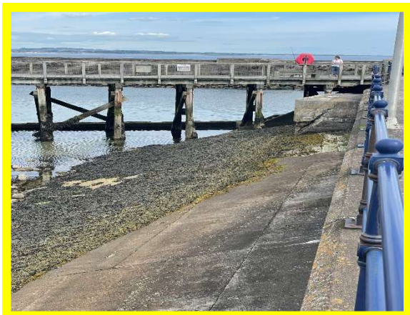
Inner face of South Pier in fair condition (/3101C02)
