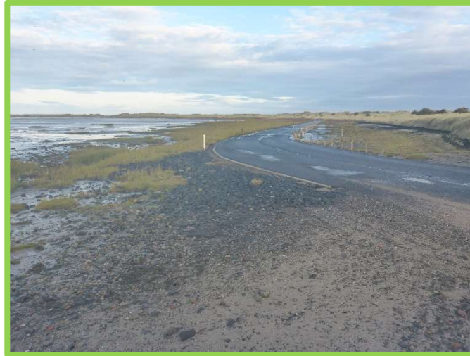
Repaired road surface and kerb at Chare Ends in 2016 (4901c01)
