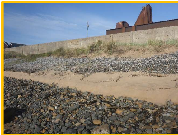
Gabions protecting very narrow strip of dunes (/4201C03)
