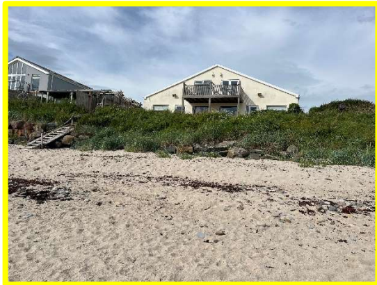
Dumped rock fronting properties at Beadnell Haven (1701C24)
