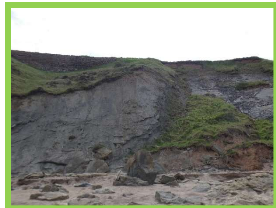
1001 c05 – 2022 no substantial change in coastal slope.
