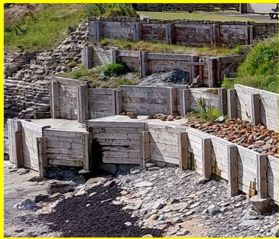
Private timber/rubble retaining defences north of Snab Point (/3301C01)
