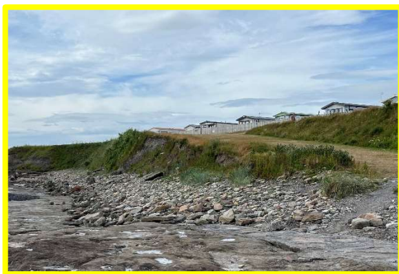
Eroding access ramp (1701C22)
