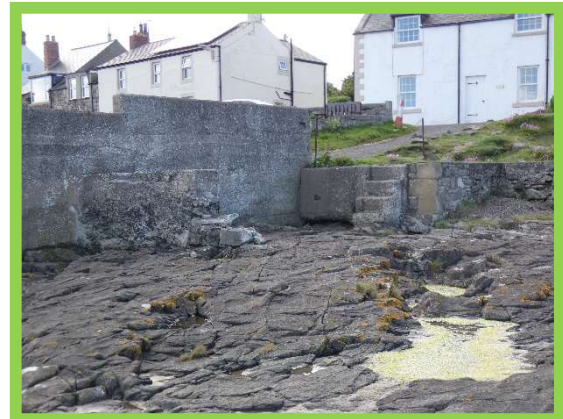
Wall and start of Pier (/2201C02 / C03)
