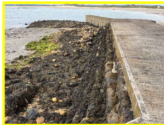
Seaward face appears in fair condition (1701C50 & 1701C51)
