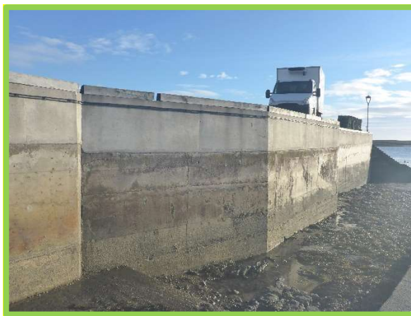
Improvement works to harbour pier (/4901c09)
