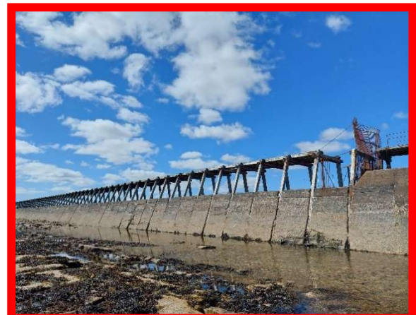
Timber deck supported by timber legs – not accessible (/4001C05)
