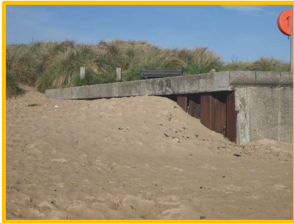
Steel sheet pile end to promenade (/4201C08)
