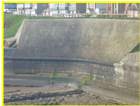
Seawall with upper brickwork retaining wall (/4401C15)
