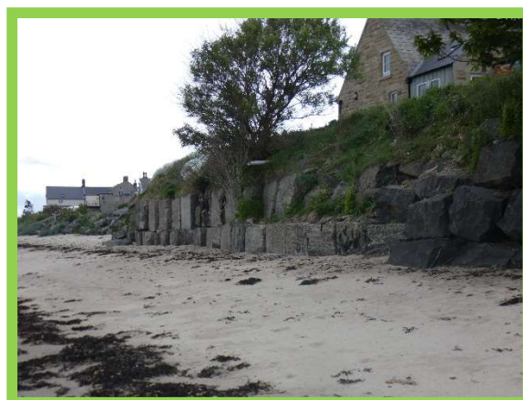
2601/C02 Block revetment, no change
