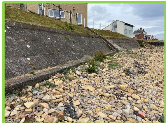
Concrete revetment in good condition, evidence of grout repairs at southern end (1701C42)
