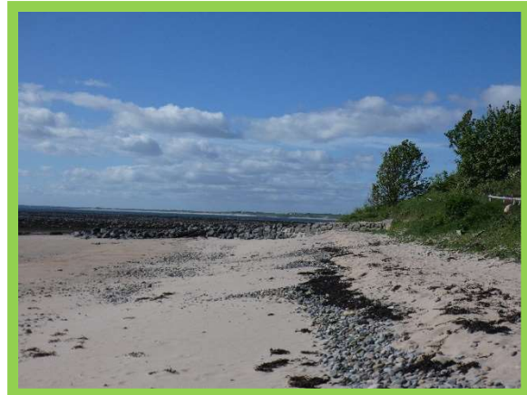
2701/C03 Timber breastwork and low masonry wall fronting property
