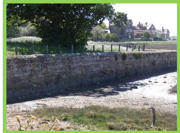
2801/C06 Masonry wall fronted by salt marsh, no change
