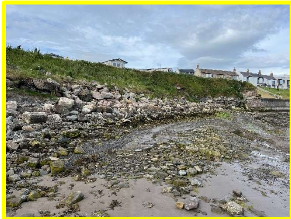
Tipped rubble slope (1701C19)
