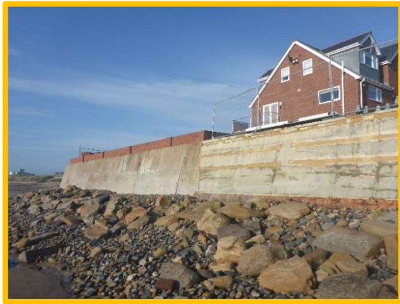
Original and extended sea walls protecting new properties (/4201C04)
