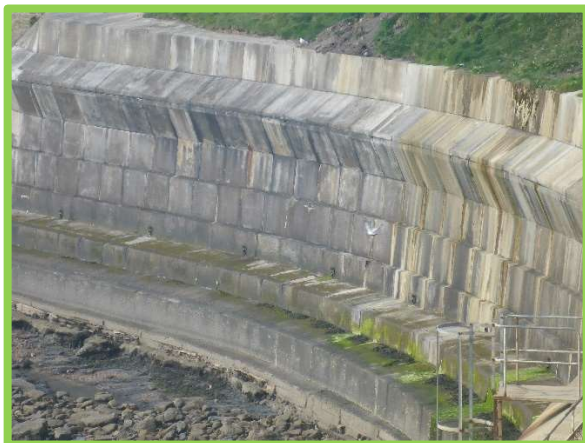
Near-vertical seawall (/4401C14)
