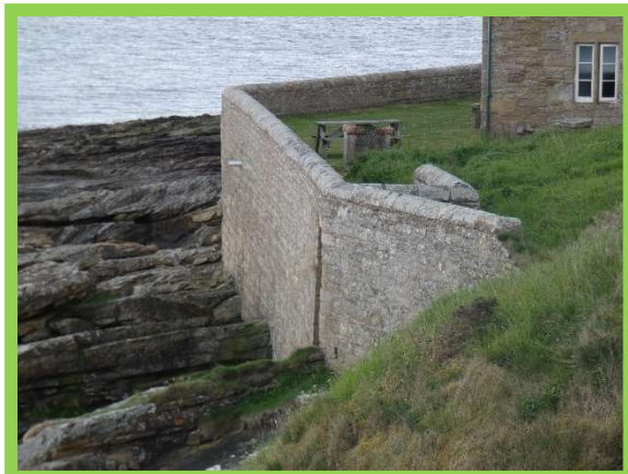
2401/C02 Bathing House wall
