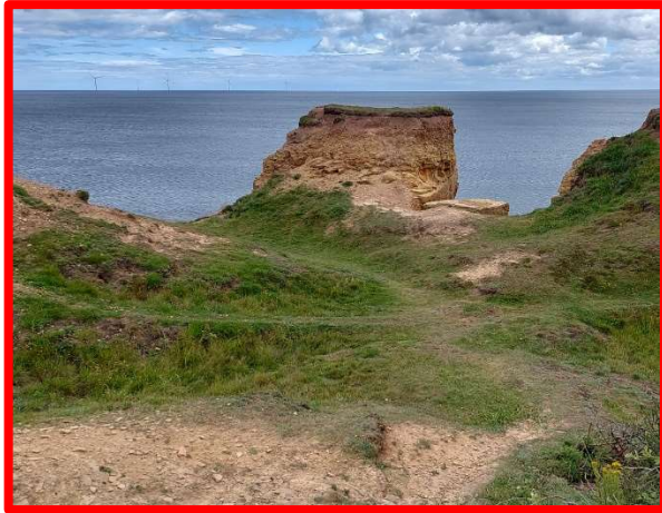
Collapsed section of Hawks Cliff (/3701C02)
