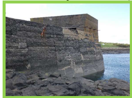
2201C11 Front face of Pier no change
