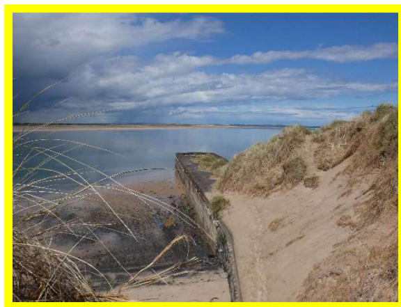
1501/C06 – South face and core of Jetty 2022
