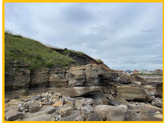
Ongoing erosion of cliffs around Dell Point (/1701C28)
