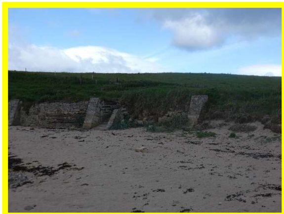
2501/C01 series of masonry walls to coastal path.
