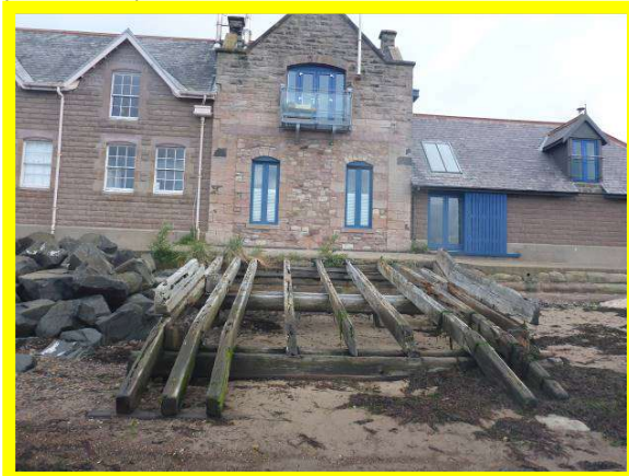
Obsolete timber slipway (/0801C05) 2020
