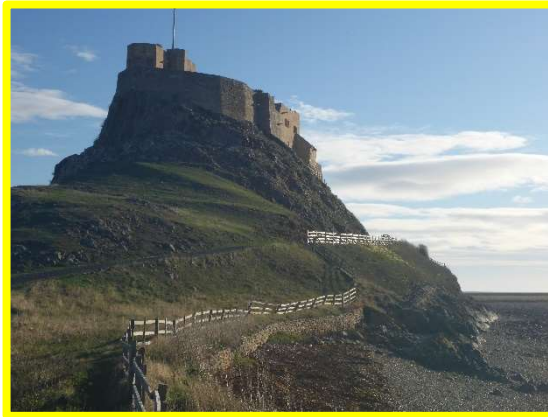
Wall And cliff below castle east of erosion matting (/4901c12-c13).
