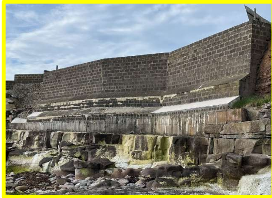
Maintenance repair works since 2020 to concrete apron and blockwork (1701C02)
