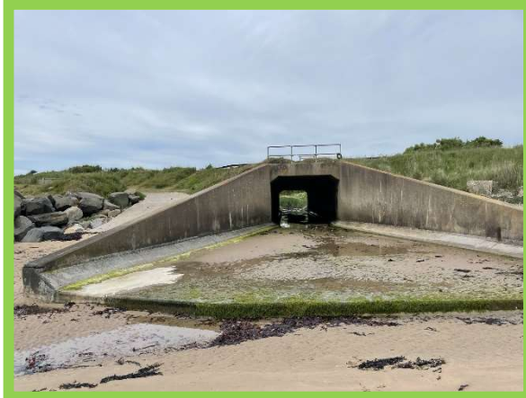
Concrete outfall and adjacent rock revetment (/3201C12)
