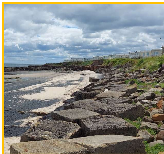
More stable central section fronting caravan park (/3501C06)
