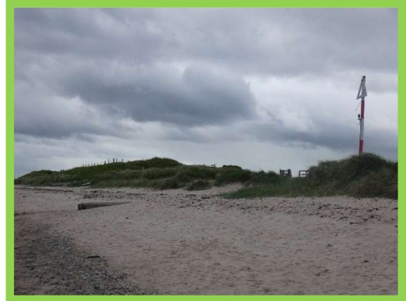
2601/C06 (southern end) Local toe growth
