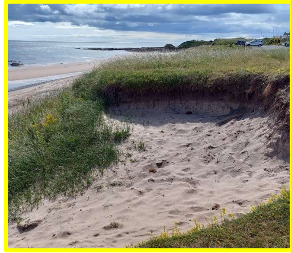
Slippage north of the car park (/3201C21)
