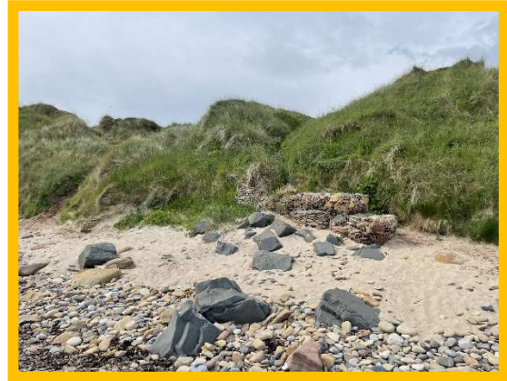
Access steps through dunes protected at base with gabions (/3101C12)
