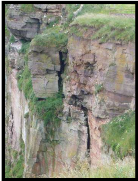
Fractured cliffs at Marshall Meadows Bay (/0601C02) - 2016
