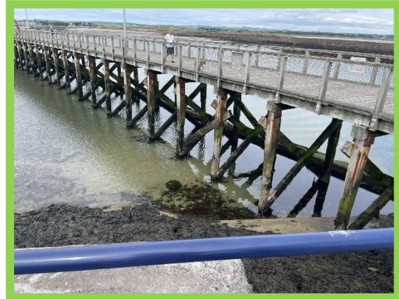
Good condition of South Jetty (/3101C11)
