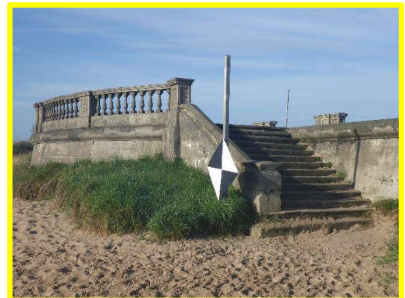
Seawall and access steps (/4201C05)
